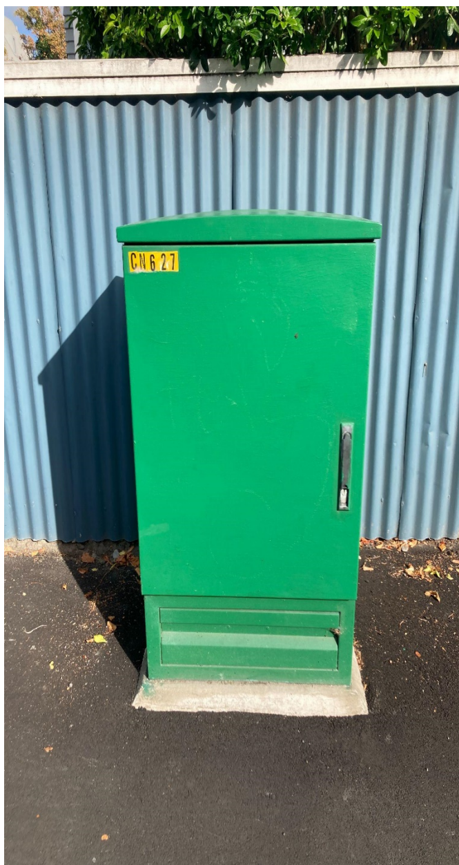
Photo four: An Enable Networks roadside cabinet. Fibre from central offices is sent to cabinets around the city. Approximately 128 customers can be fed from a single cabinet.
